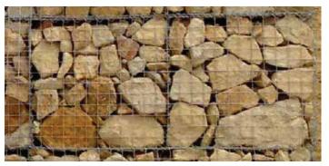
Above (Option 2): Gabion wall at neighborhood monument. Rotate stones when placing in basket so face of stone is flat to basket, minimizing voids along face of wall.
